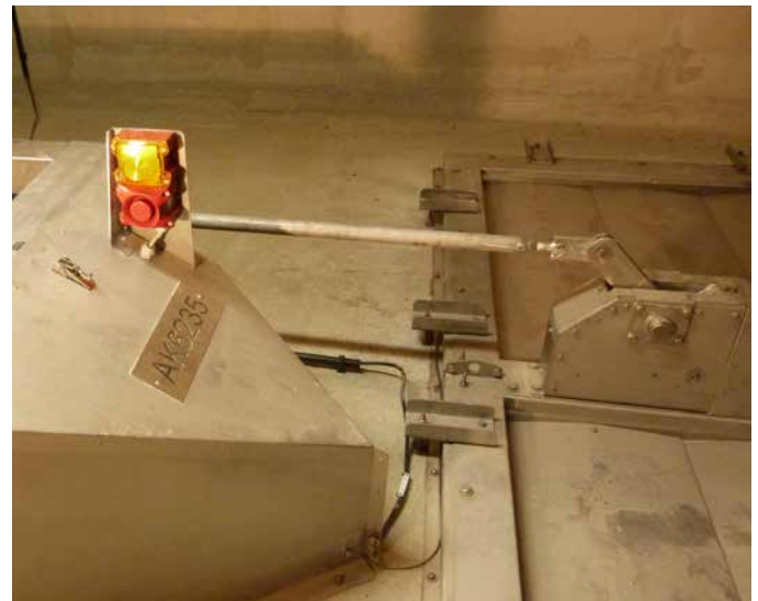
There is a ventilation damper installed every 100 meters in the two ducts along the length of the tunnel. If fire breaks out, the Pfannenber signaling devices will issue a visual and audible alert. Smoke extraction cannot start until confirmation has been received that evacuation is complete.
