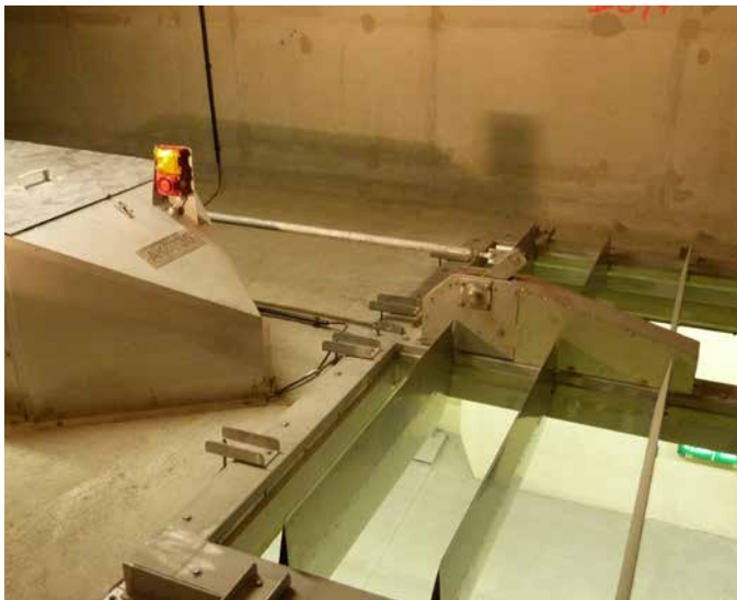
Open ventilation damper in the Gleinalm Tunnel showing the traffic tunnel below. There are around 80 dampers installed in each of the two ventilation ducts which will also act as controlled smoke extractors in the event of a fire.
