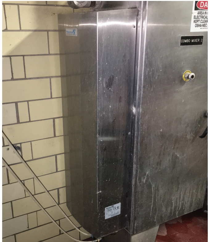
Fig. 4: Pfannenberger's PWS unit installed on enclosure
