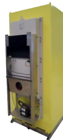
Fig. 3: Electrical enclosure with Pfannenber DTGT cooling unit without top cover
