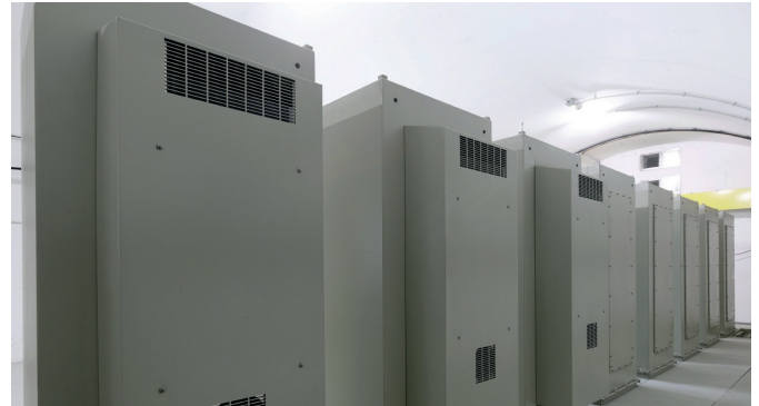
Fig. 2: Swibox electrical enclosures in cross passage of Lötschberg Tunnel
