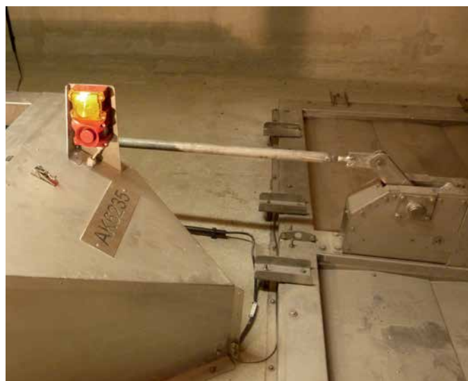
There is a ventilation damper installed every 100 meters in the two ducts along the length of the tunnel. If fire breaks out, the Pfannenberg signaling devices will issue a visual and audible alert. Smoke extraction cannot start until confirmation has been received that evacuation is complete.
