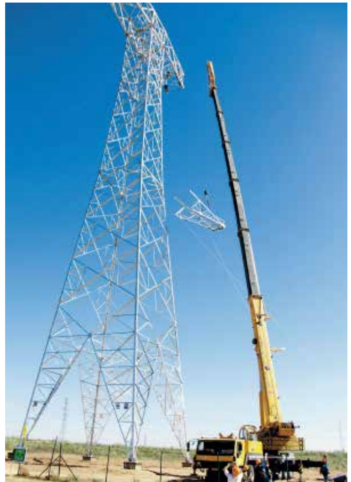
UHVDC line under construction
