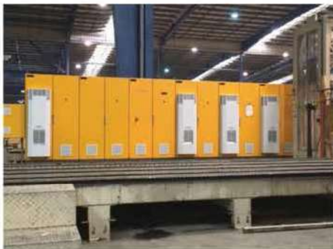
The electrical enclosures for the packaging line after being refitted with DTI cooling units.
