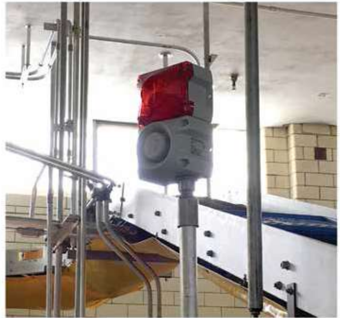
Pfanneneberg The PA X 1-05 Flashing Light Sounder in the inspection line
