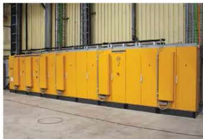
New switchgear cabinet for a short-cycle press for flooring manufacture, equipped with air/water heat exchangers from Pfannenberg.
