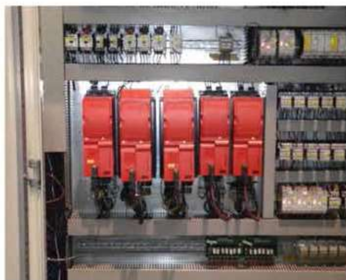
Very dirty frequency converters before cleaning (above). The cleaned switchgear (below) was put back into reliable operation for the packaging line.
