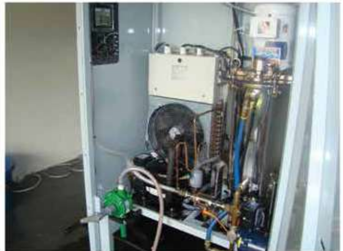
Pfannenberg open-frame chiller inside packaged Ferrator.
