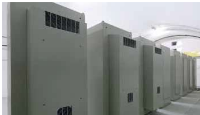
Fig. 2: Swibox electrical enclosures in cross passage of Lötschberg Tunnel
