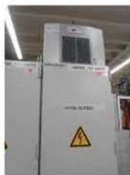
DTT-top-mounted cooling units reliably prevent the penetration of condensate into electrical enclosures
