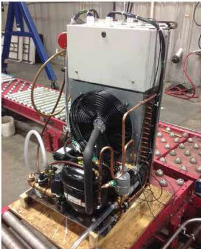
Pfannenberg open-frame chiller on factory production line.
