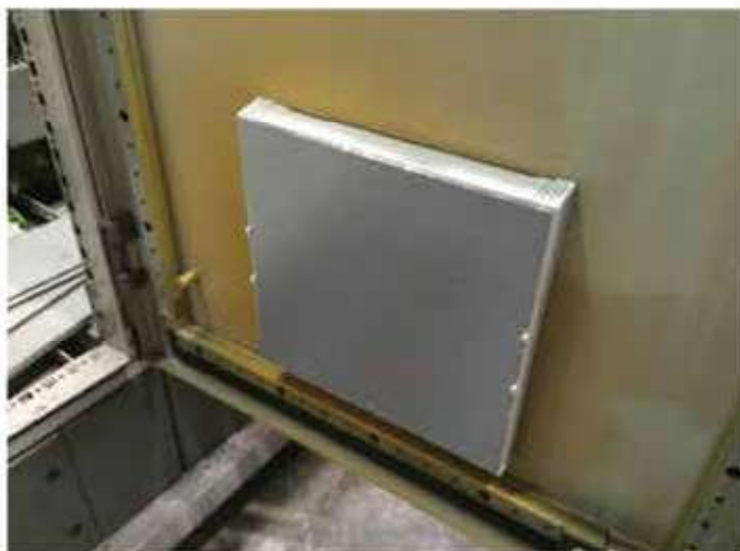
The filter fans from Pfannenberg are fully sealed so that no air can enter them.
