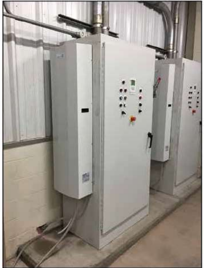
Pfannenberg air-to-water heat exchange on a lift pump control panel at a wastewater treatment facility.
