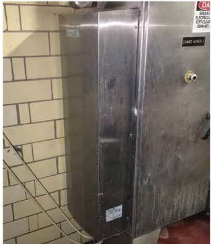
Fig. 4: Pfannenbergs' PWS unit installed on enclosure
