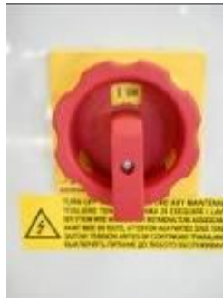
Picture 16 – Main switch ON
