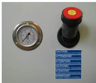
Picture 9 – Example of filling point
