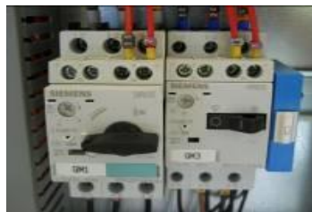
Picture 8 – Circuit breakers OFF
