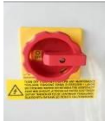
Picture 7 – Main switch OFF
