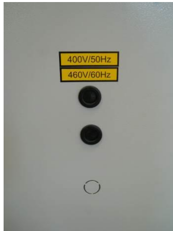
Picture 13 – Electrical connections
