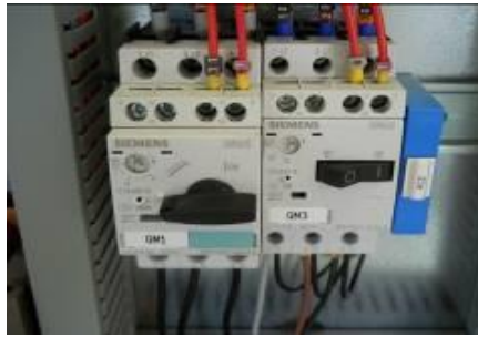
Picture 15 – pump breaker On
